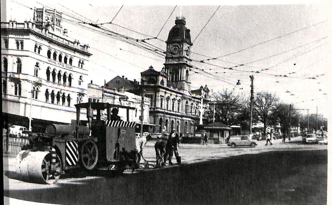
Trackwork in Sturt St. August 1966, using the locally built Jelbart oil roller (now at TMSV
