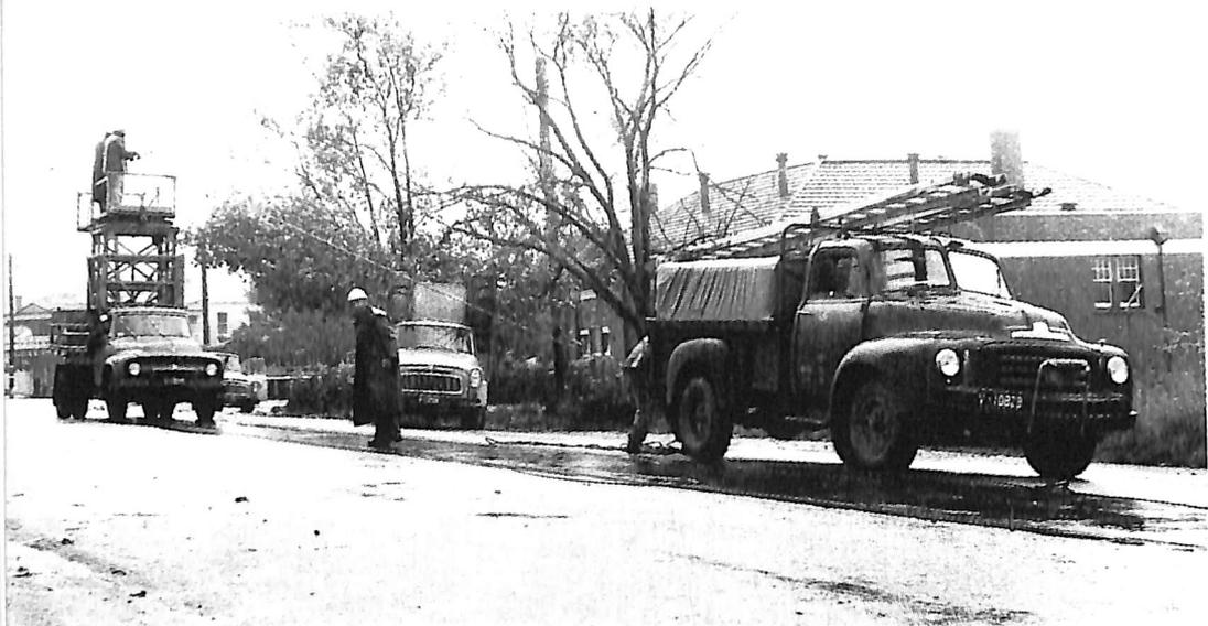
Often repairs to the Overhead were necessary, and often after a storm. The overhead crew repair fallen wires, possibly after tree branch fell in Lydiard St. North during April 1965.
